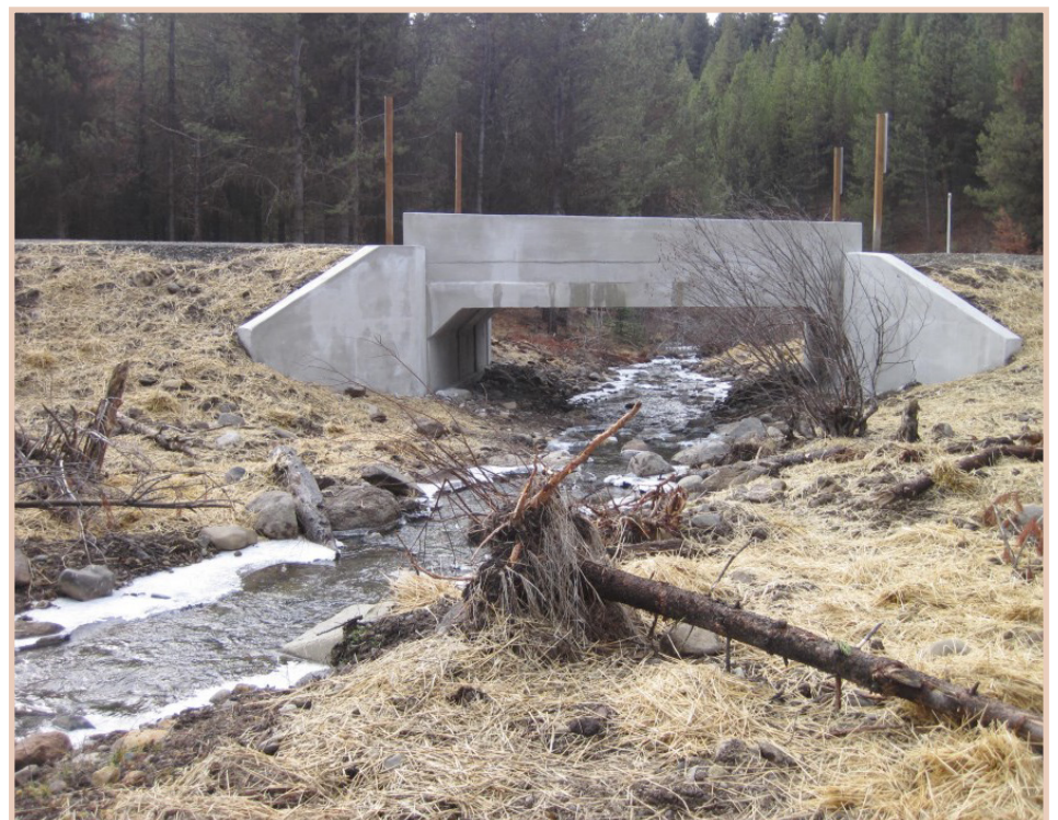
AFTER: The project replaced the culvert with a concrete bridge. The channel through the bridge simulates natural stream width and gradient (courtesy of Joe Platz).
