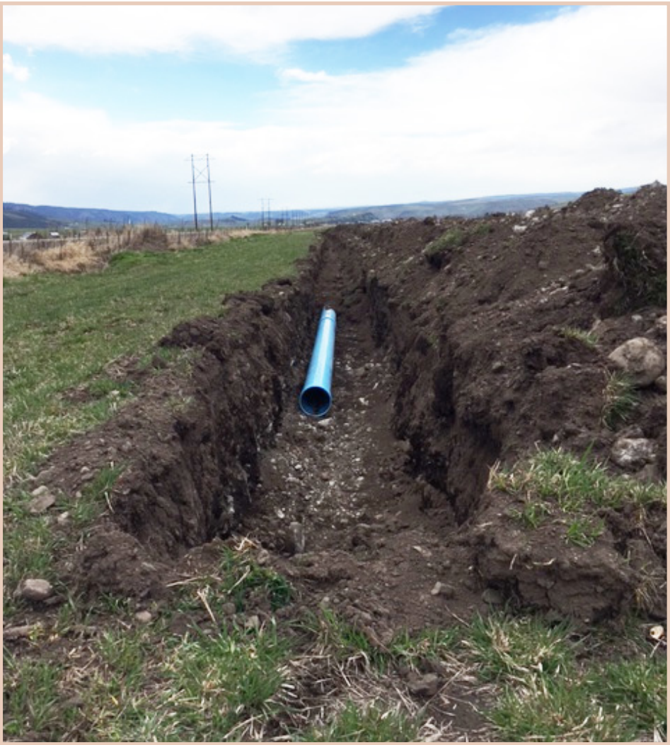
Excavated trench for mainline, April 2017 (courtesy of Aaron Maxwell).
