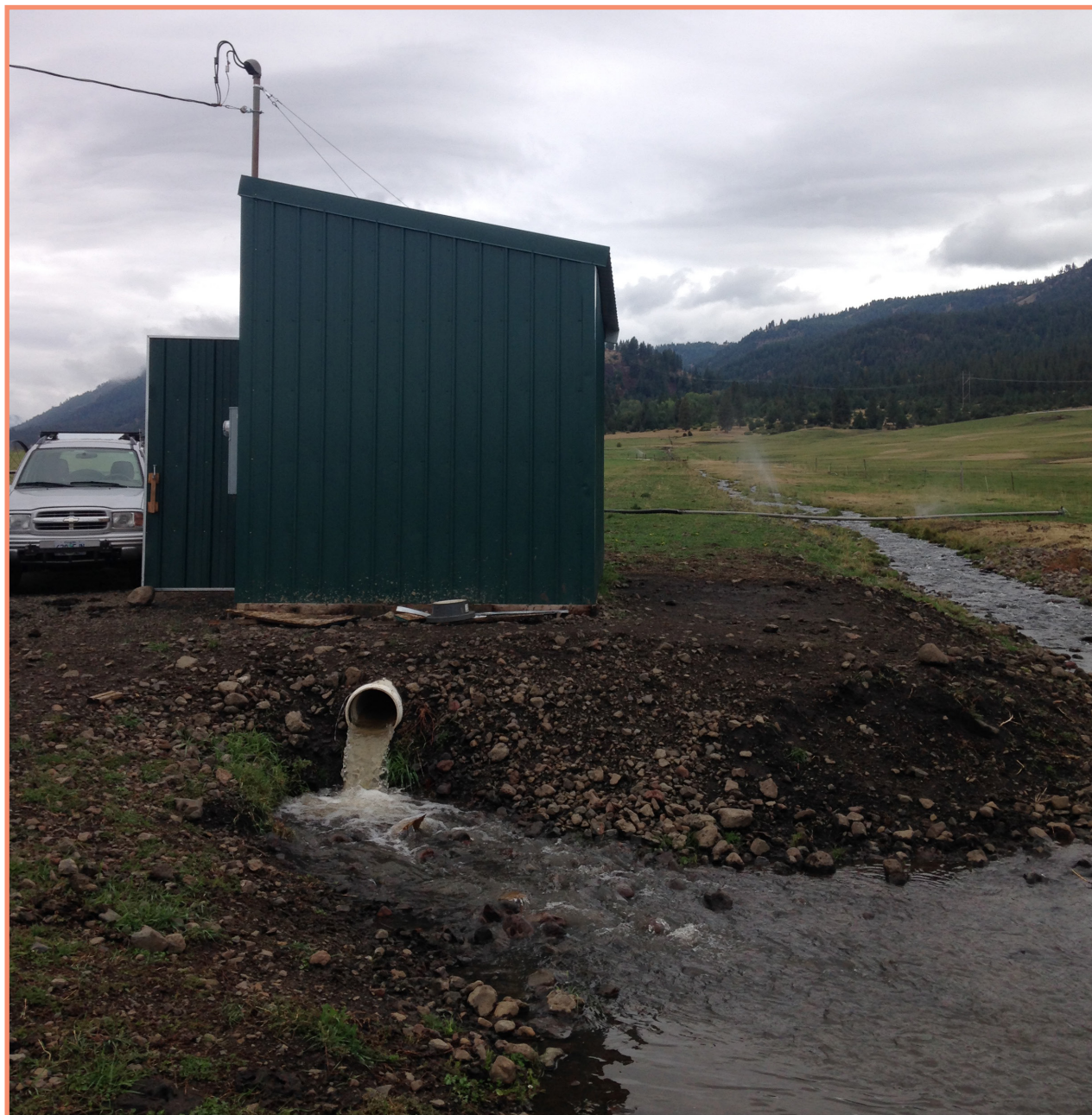
Vern Spaur’s second hydro station uses water discharged from the first station to generate power before dumping the water back into the irrigation ditch (courtesy of Malcolm Moncheur).
