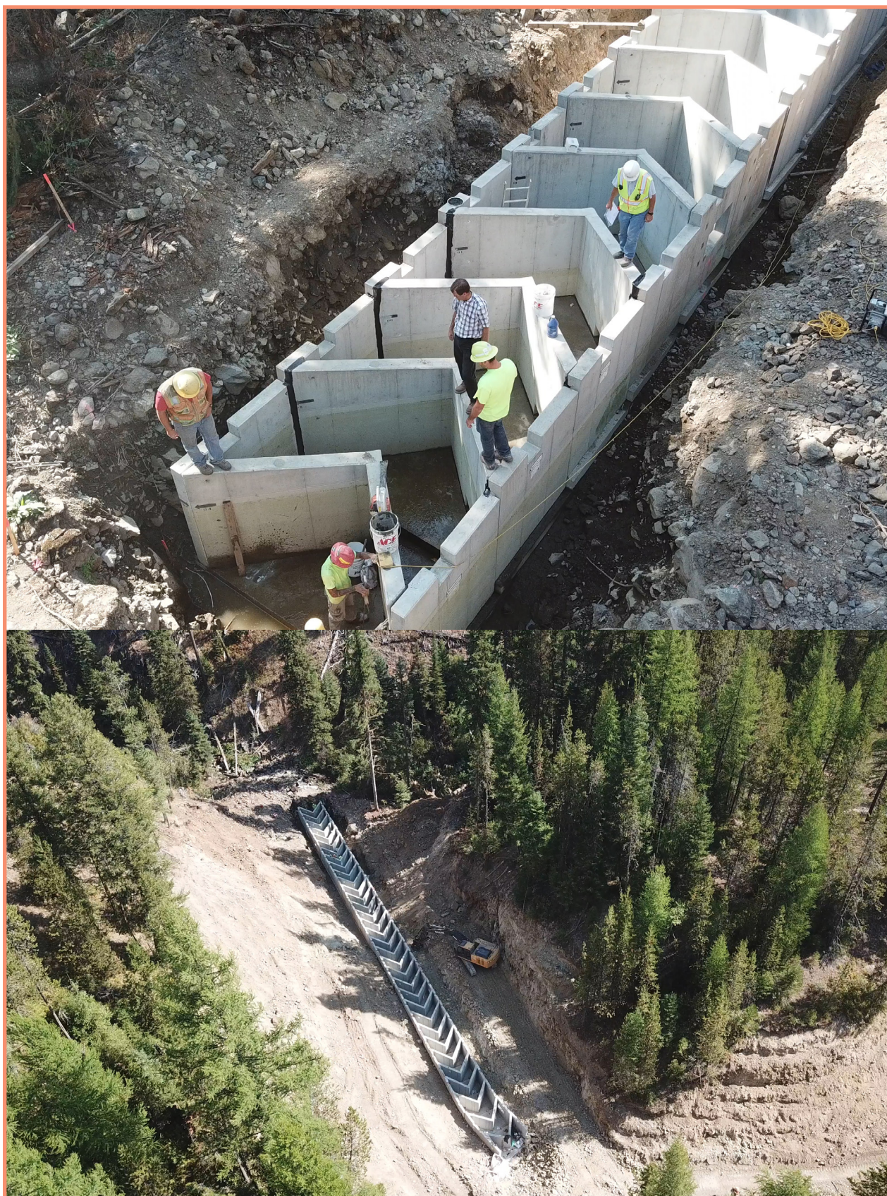
Individual precast concrete fish ladder steps being installed in the middle of the dam spillway (courtesy of Anderson Perry & Associates Inc.).
