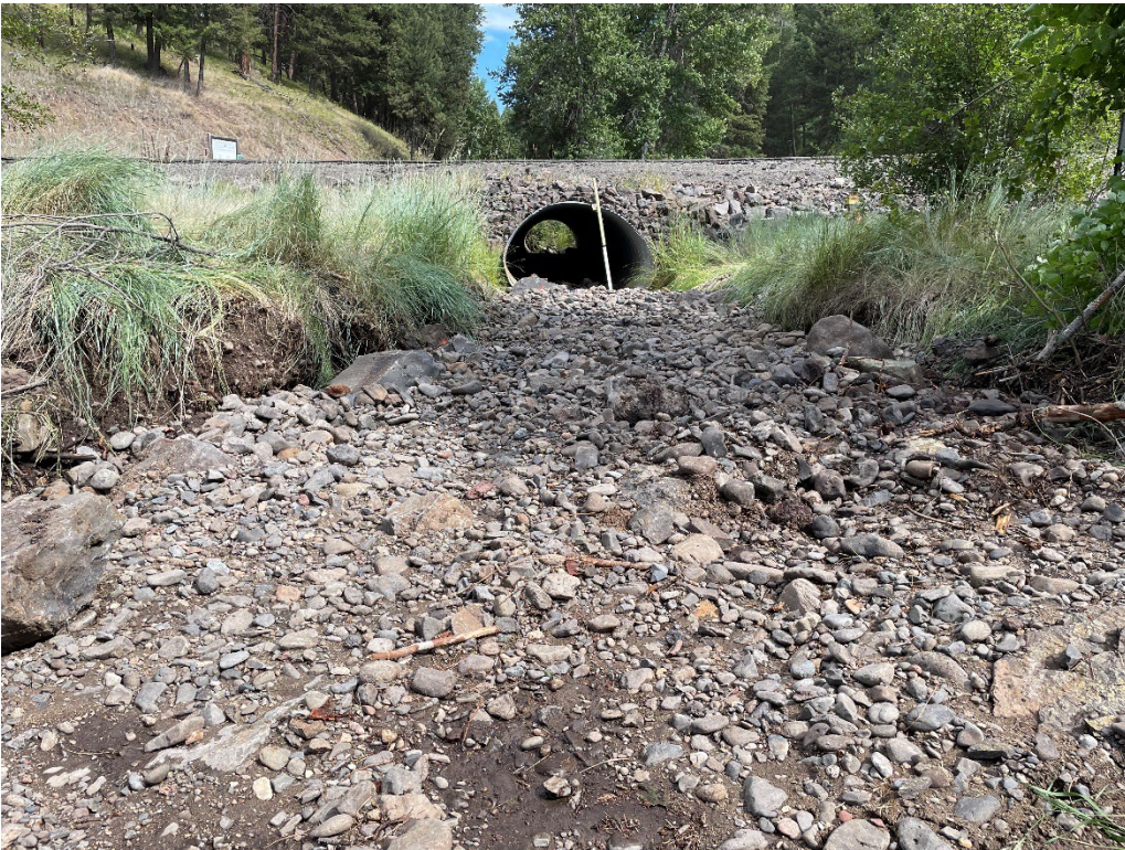
Figures 5 and 6. Construction of the Warm Springs Creek alluvial fan and channel.
