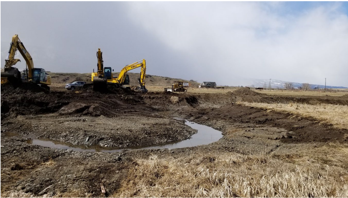
Looking downstream at the same reach of Side-channel 1 during construction on 03/29/2021. Channel was dug “in the dry” outside of the in-water work window.
