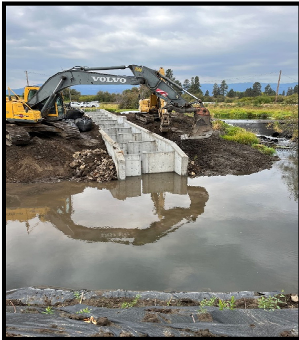
Figure 4. Huber Dam Fishway, installation of surrounding rock apron.
