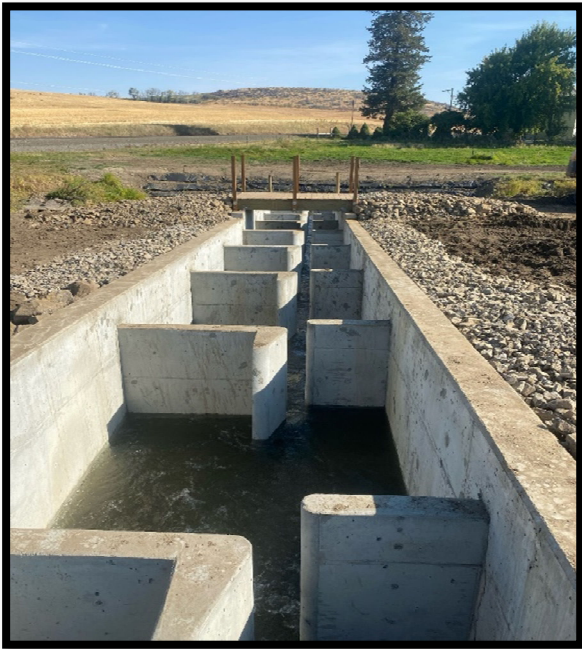
Figure 3. Huber Dam Fishway activated with flow.
