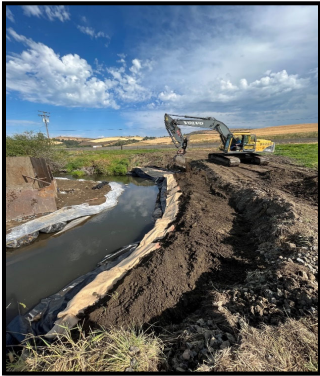
Figure 5. Construction of encapsulated soil lift.
