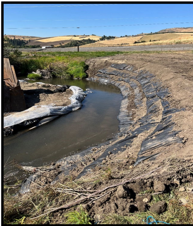
Figure 6. Completed encapsulated soil lift.
