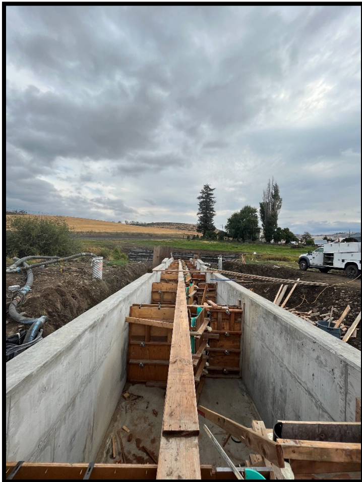
Figure 2. Huber Dam Fishway construction, weir wall forms.
