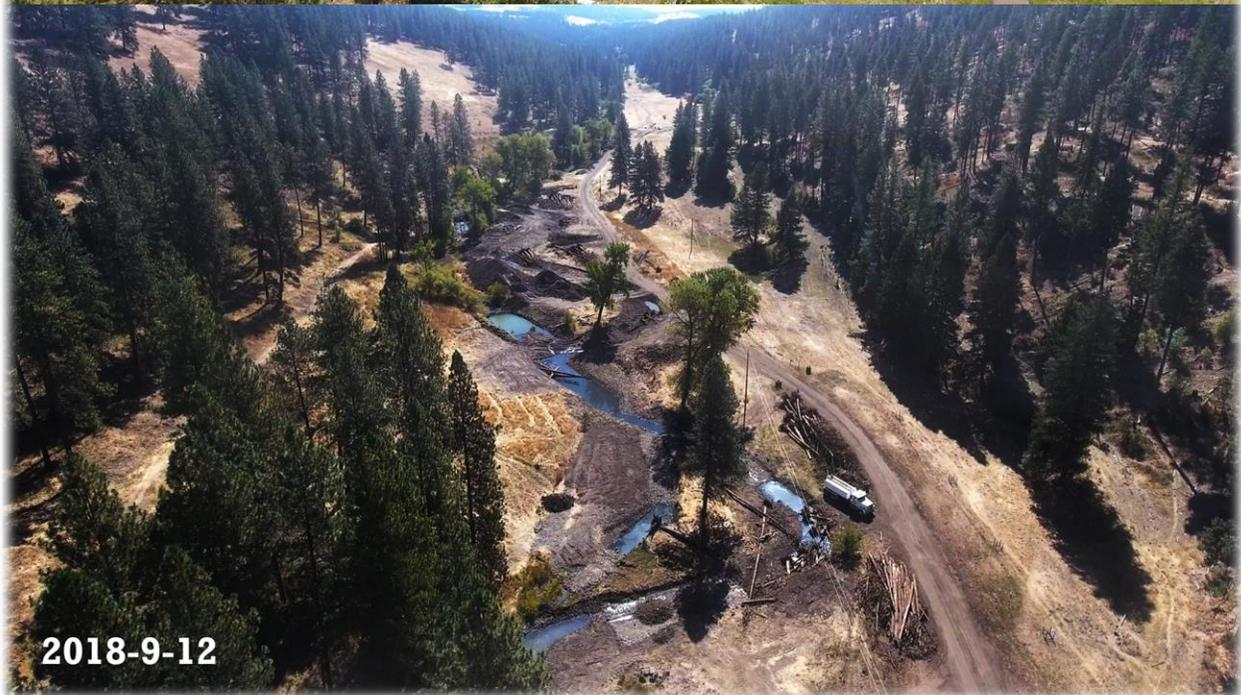
*A tributary to the Upper Grande Ronde and an important steelhead stream, Rock Creek is on private land. Prior to restoration, Rock Creek exhibited high width to depth ratio and was incised throughout most of its length. CTUIR Habitat Program, working with the landowner, improved sinuosity and floodplain connection as well as narrowing the channel. This project was funded primarily by BPA and will be completed in 2019. Photos by Connor Stone (GRMW).*
